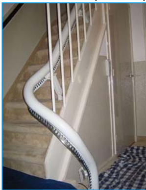
Figure 2-8: Spirale et palier vertical
